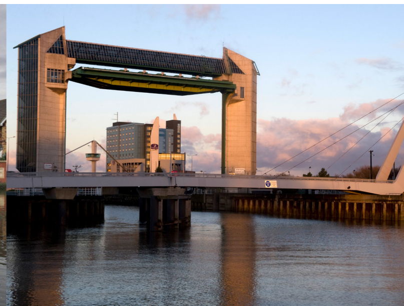
Figure 4: Tidal Surge Barrier, Kingston upon Hull - photo by Sean Spencer
