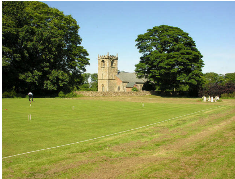
Rowley today: St. Peter's Church, Rowley, East Yorkshire (source: http://en.wikipedia.org/wiki/Rowley,_East_Riding_of_Yorkshire )
