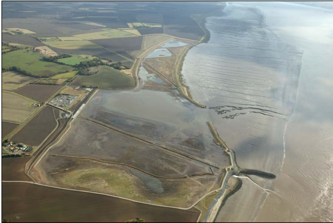
Plate A: Aerial view of Paul Holme Strays site following the embankment breaches (October 2003, Environment Agency)
