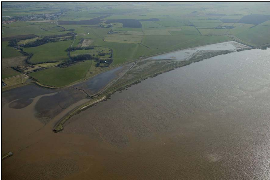
Plate B: The site in the third year post-breach (January 2006, Environment Agency)
